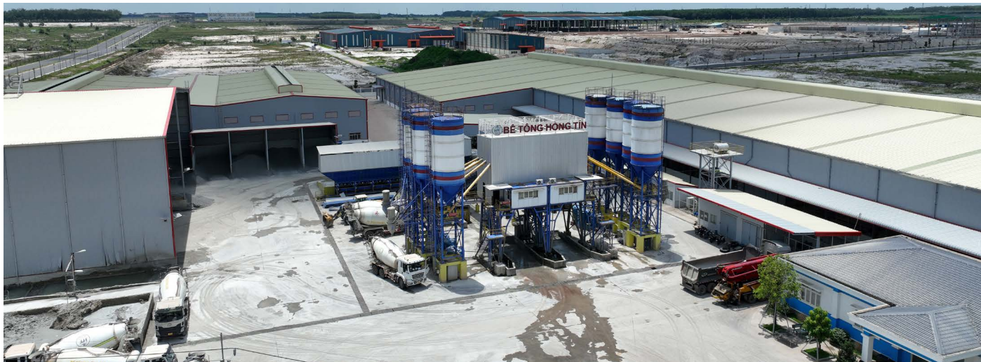
Hong Tin Concrete Plant - Binh Phuoc Location: Becamex Industrial Park – Binh Phuoc, Chon Thanh District, Binh Phuoc Province Size: 13.264 m 2 Capacity: 3 x 120 m 3 /h
