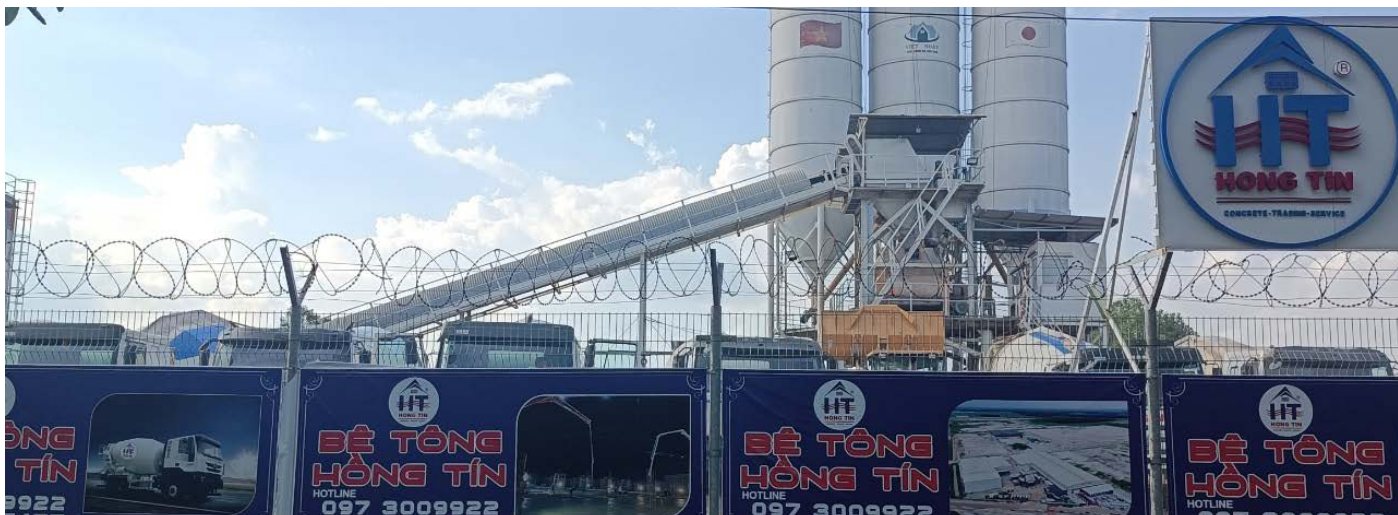
Hong Tin Concrete Plant - Tram Phu My Location: Phu My 1 Industrial Park, Phu My Town, Ba Ria - Vung Tau Province Size: 5.500 m 2 Capacity: 120 m 3 /h
