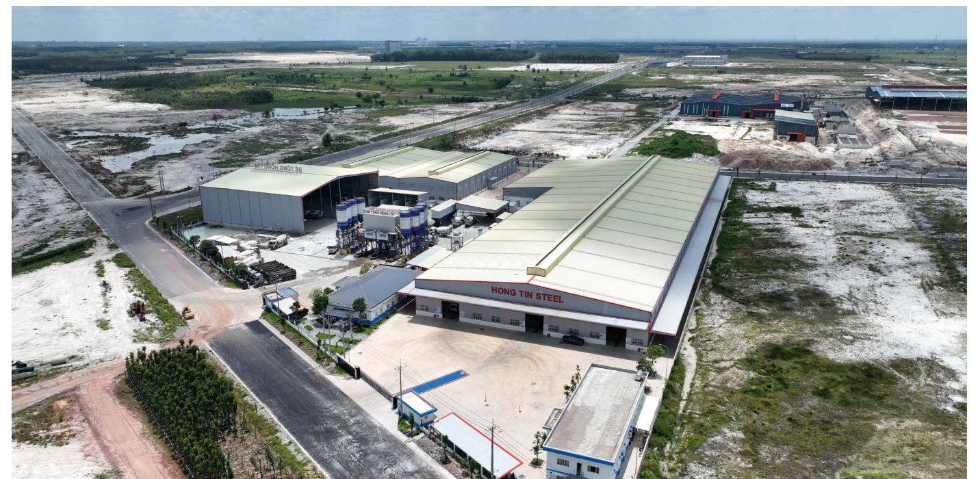
Hong Tin Structural Steel Plant - Binh Phuoc
