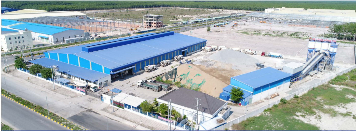
Hong Tin Concrete Plant - Binh Duong Location: Tan Binh Industrial Park, Bau Bang District, Binh Duong Province Size: 20.000 m 2 Capacity: 2 x 120 m 3 /h
