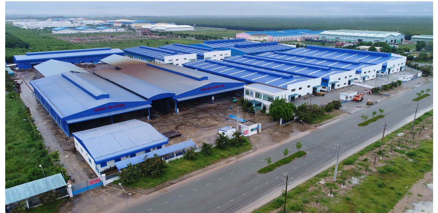
Hong Tin Structural Steel Plant - Binh Duong
